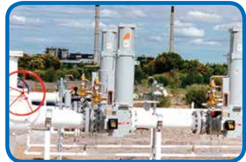
Figure 13 - Becker RPSR Actuated Control Valves in Power Plant A Becker RPSR actuated control valve is used to provide primary pressure regulation and overpressure protection (monitor regulators) on a feed to a gas-fired power plant. The RPSR shown here are equipped with Becker Model HPP-SB High Pressure Positioners to provide maximum speed of response combined with optimum accuracy.
